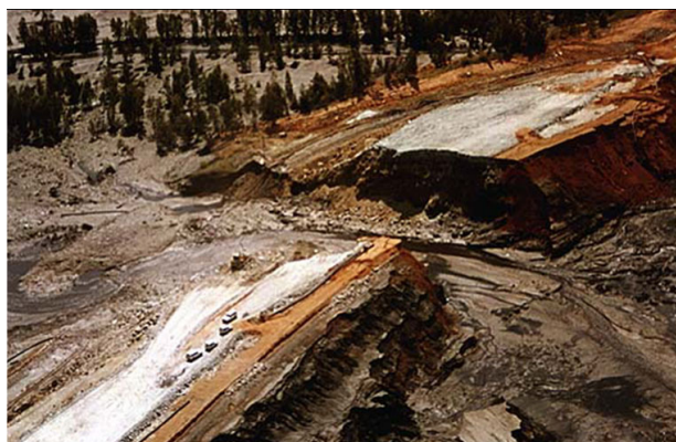
Image 1: Aznalcollar (Spain). Failure of tailings dam retaining wall, 25 April, 1998.
