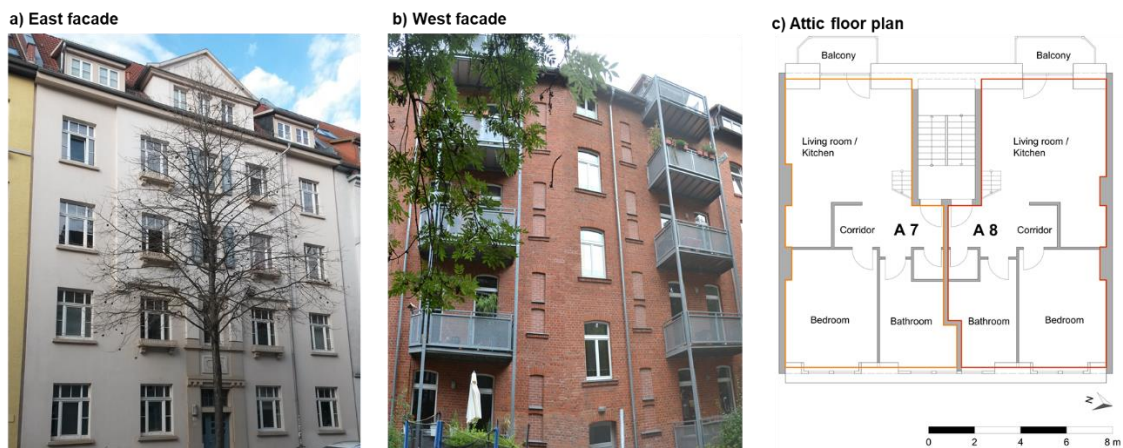
Figure 2: a) East-facing and b) west-facing façade of the GZH building; c) floor plan of the attic floor of the GZH.
