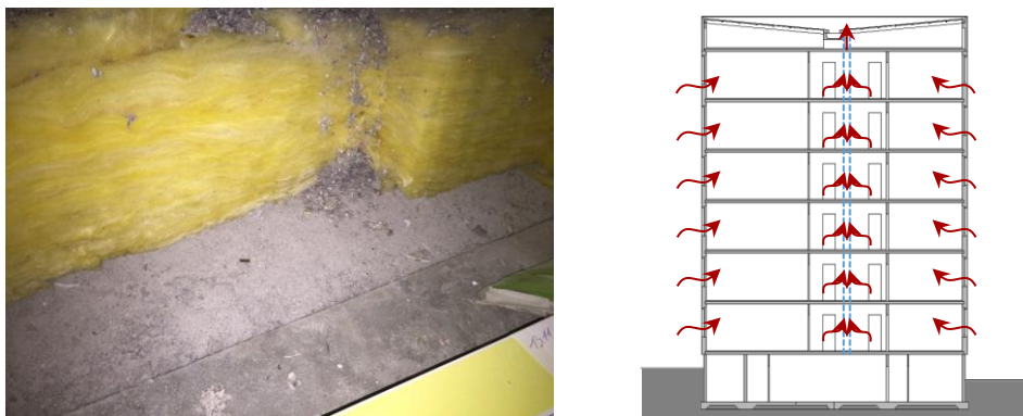
Figure 9. left: additional layers of floor screed and mineral wool insulation. Picture: © Zweinert (2020), right: section with central ventilation system to support air change during night. Picture: © Schiela (2019)
