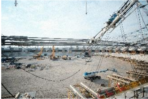
Figure 7 The lifting process
