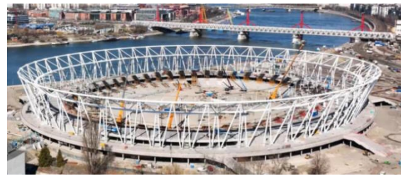
Figure 9 The cable lifting final stage
